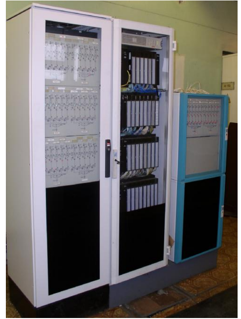
The photo of the sample delivery system “Kontur” and the control box with the “Ge Fanuc” controllers. This system is developed for Kaztsink Corporation (Kazakhstan).
